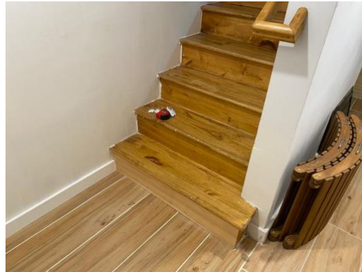
Figure (10) – Staircase landing to basement
